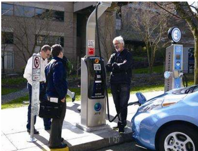
Figure 15: RAPIDAS / Kanematsu 208 volt Battery Backed Fast Charger on Portland’s “Electric Avenue” 17
