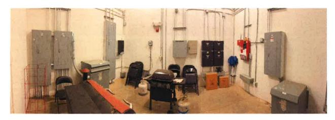
Panoramic View of Electrical Room in Building A. Indicative of general arrangement of electrical service in all buildings depending on size. Also shown control panels for WinDSX RFID system (Black) present in all buildings on campus. Fire Suppression Main Panel (Red)
