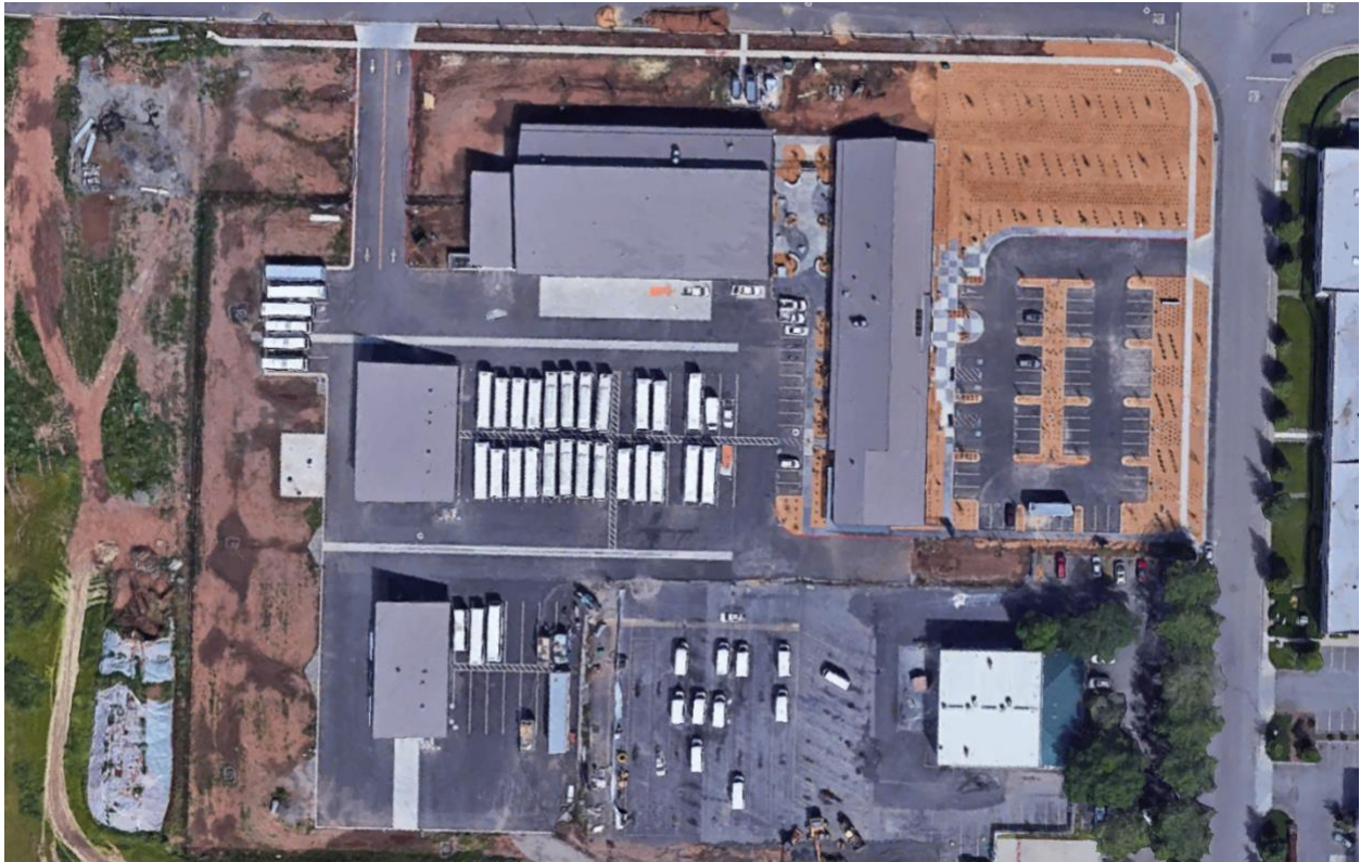
Figure 3 - Butte Regional Operations Center
