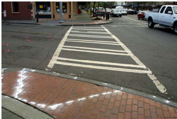
ADA requirements were often originally met in haste without proper alignment of paths. Many municipalities are now correcting these placements.
