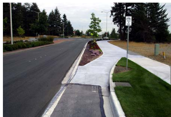
Since vehicles are slowing to 20-25mph, bicyclists entering the roundabout can either take the lane and proceed through the circle or exit and cross at the pedestrian crosswalk. Sidewalks should be wide enough to prevent conflicts with pedestrians.
