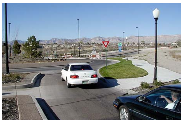
One lane roundabouts are easy to cross since vehicle speeds are low, the crossing distance is shortened to less than 14-feet and the pedestrian only has to deal with traffic from one direction. Drivers are also more likely to yield to pedestrians at these slower speeds.
