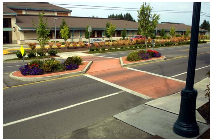
Detail of the mid-block islands/crossings proposed along Nord Avenue. The angled crosswalk through the island improves safety by forcing pedestrians to look in the direction of oncoming traffic.
