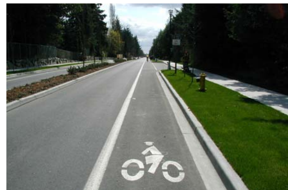
This rebuilt street in University Place, WA demonstrates some of the features of a complete street: An ample and well-marked bicycle lane, a planter strip and a 5-foot sidewalk. The travel lane is 10 feet wide, the bicycle lane is 6 feet.
