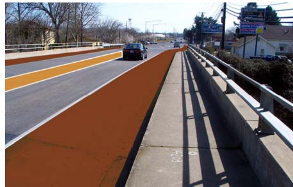
Speeds across the Lindo Channel Bridge can be moderated by colorizing the bicycle lane and a narrow median. The bicycle lane provides a refuge for pedestrians on the narrow sidewalk.
