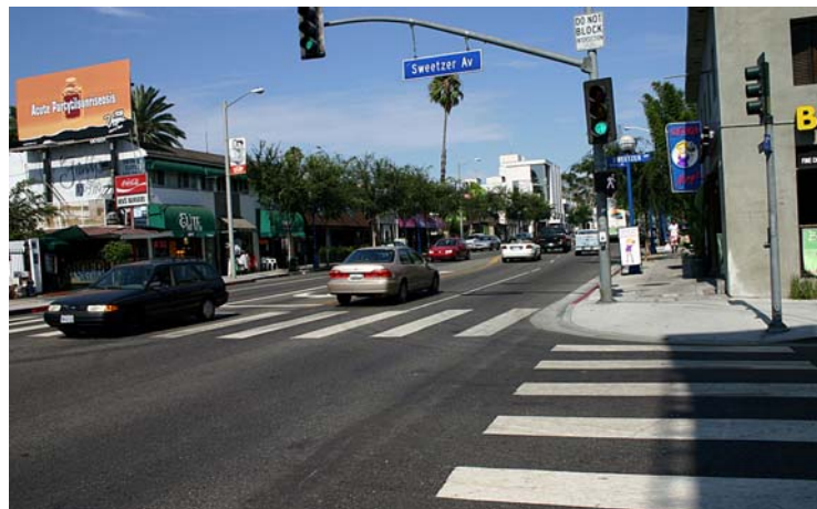
Complete streets include high-visibility crosswalk markings such as these on Santa Monica Boulevard in West Hollywood. Some cities use a lower maintenance “piano keys” design that spaces the lines so that vehicle wheels straddle them.
